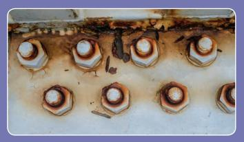
**Spot Treatment of Crevices:** Use the TR2200HS Penetrant/Sealer for spot-treating crevice corroded and pack-rusted connections directly or as part of a total structure anti-corrosion solution. The HRCSA penetrant will infiltrate deeply inside corroded connections via pressure and capillary action. The TR2200HS penetrant/sealer has also been shown to free up corrosion frozen bearings.
